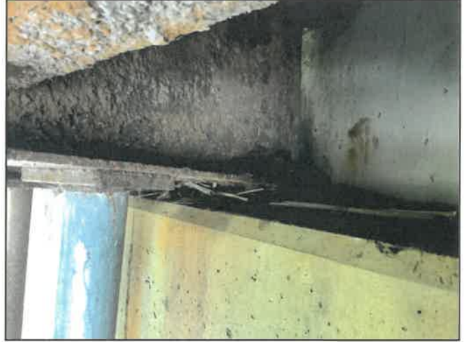
Beam 2 abutment 2 end
