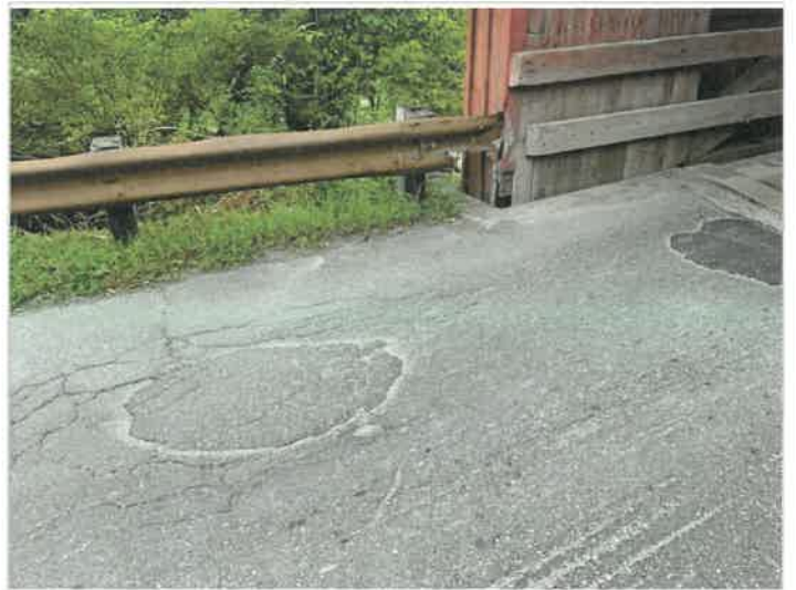
Abutment 2 transition rail
