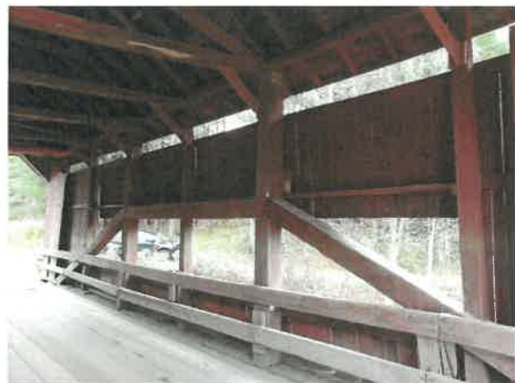
West Queenpost Truss
