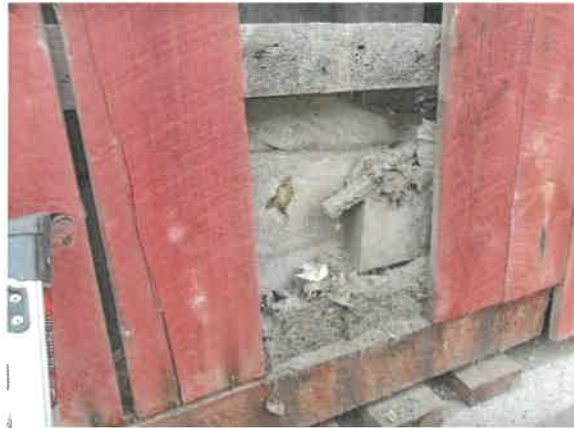
North End of the East Truss Bottom Chord to Diagonal
