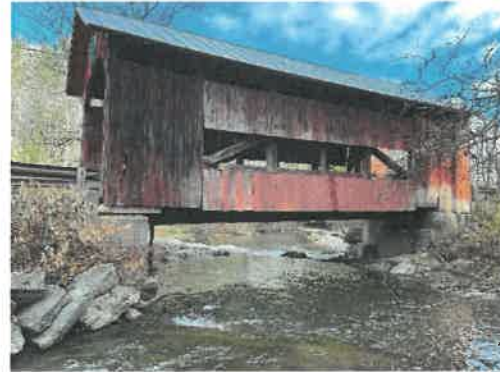
Upstream Elevation Looking East
