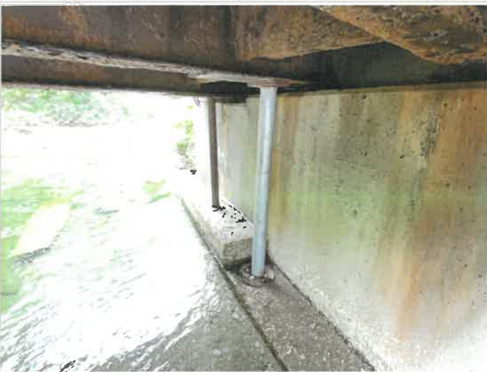
Beam 2 abutment 2 end
