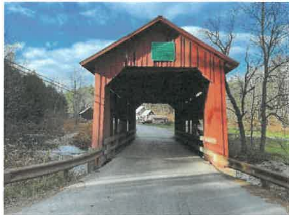
South Portal Looking North
