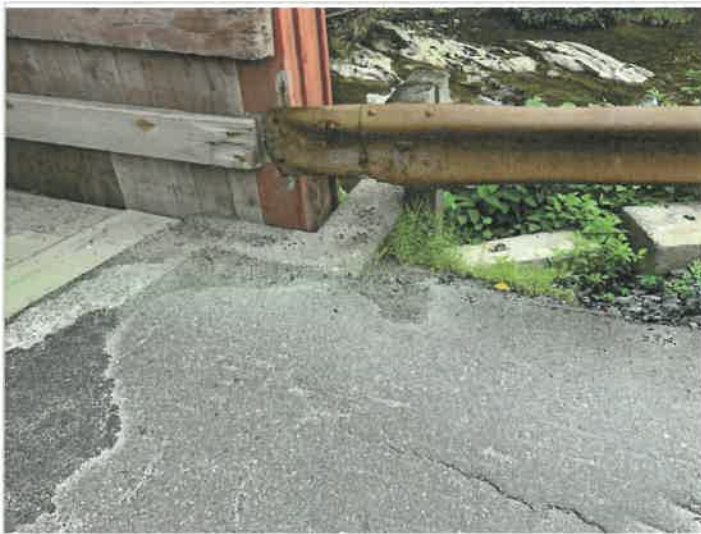
Abutment 2 transition rail
