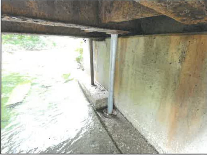
Abutment 2 beam ends
