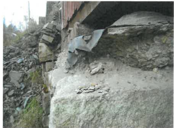
West Abutment Beam Seat
