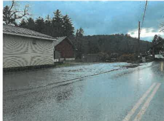
Commercial Drive at South Approach
