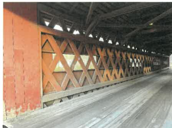
North Truss Looking East
