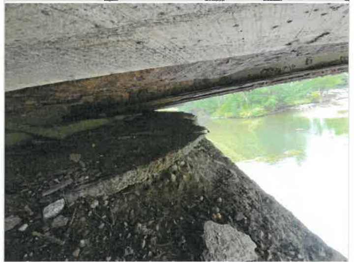
Abutment 1 beam ends
