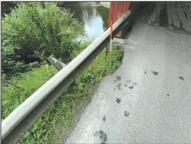
Upstream abutment 1 shoulder area
