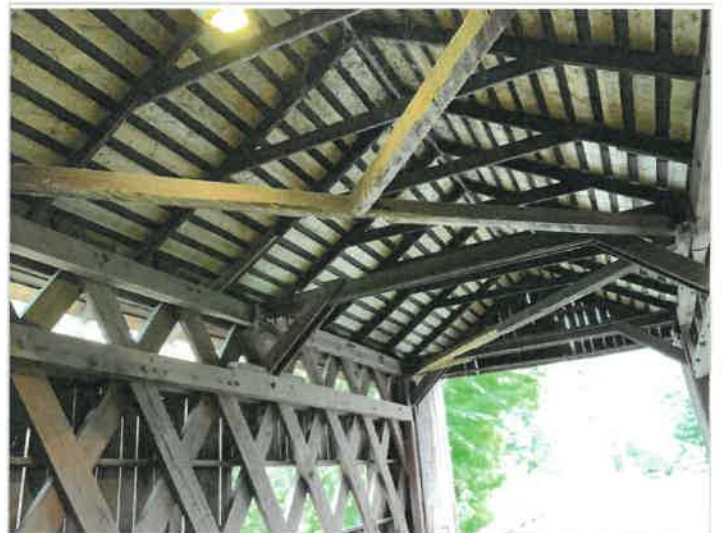
Lateral cross bracing
