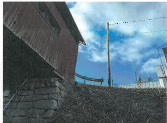
Guy Wire Attached to NW Corner of Bridge
