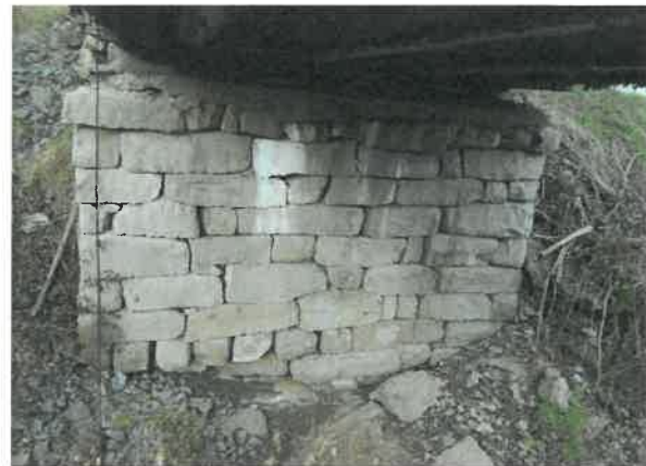
West Abutment Elevation
