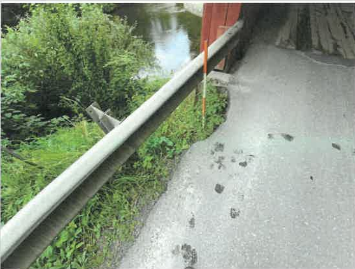
Upstream abutment 1 shoulder area
