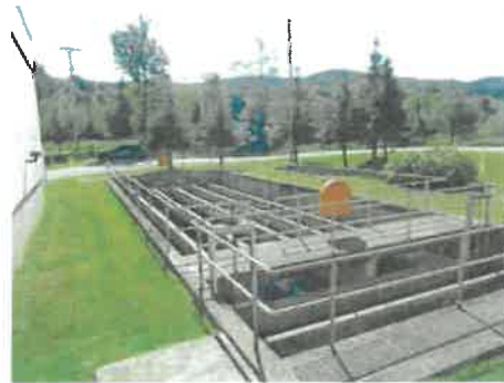
Chlorine Contact Chamber
