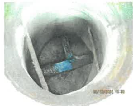
No ID – Wall + Water St.
