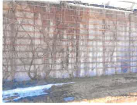
SBR Tank Wall
