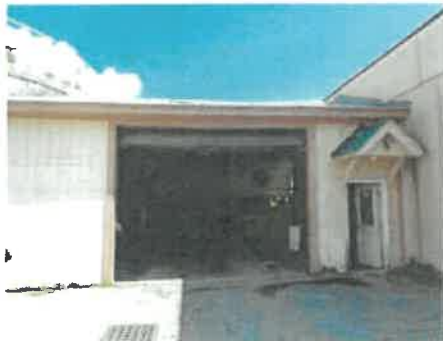
Control Building Entrance
