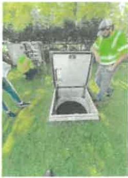
Pump Station Pit
