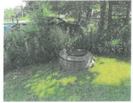
Pump Station Manhole
