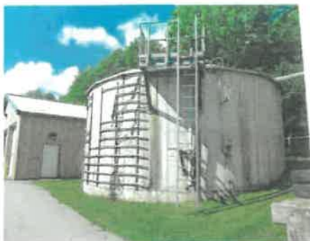
Aerated Sludge Storage Tank No. 2
