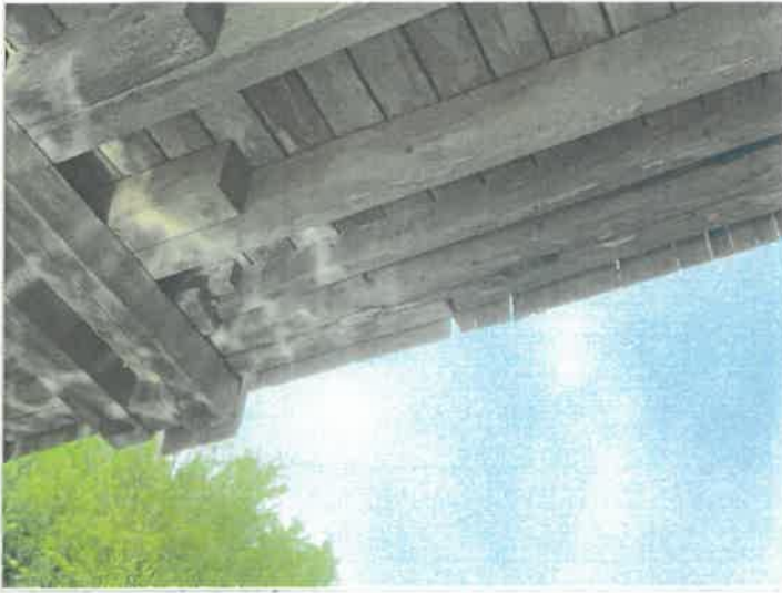
Downstream bottom chord key slot block abutment 1 end
