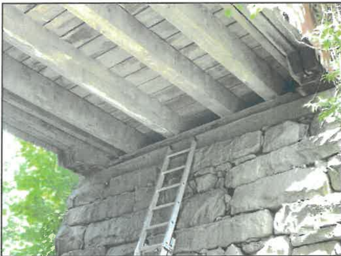
Abutment 1 bearing seat beam
