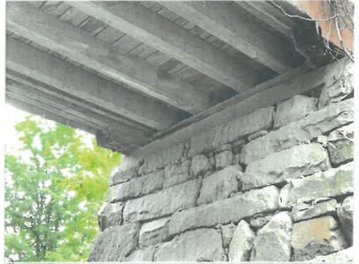
Abutment 1 stringer bearing beam
