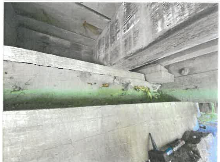
Abutment 2 bearing seat beam downstream end
