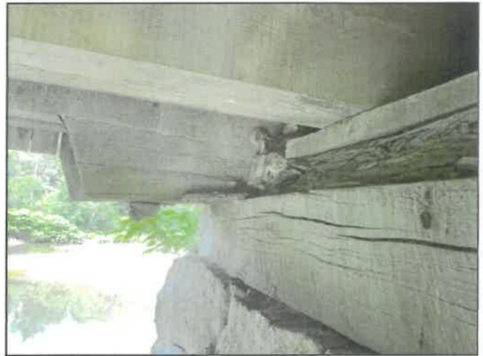
Abutment 1 downstream bolster beam bearings
