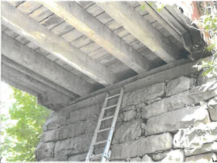
Abutment 1 bearing seat beam
