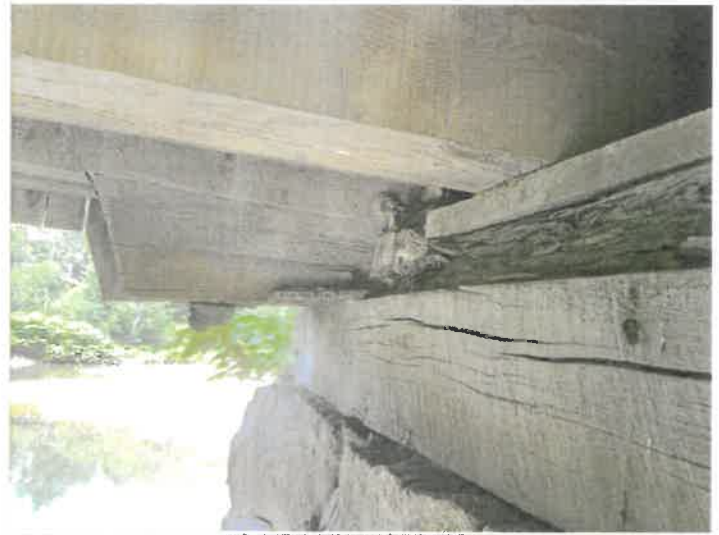
Abutment 1 downstream bolster beam bearings
