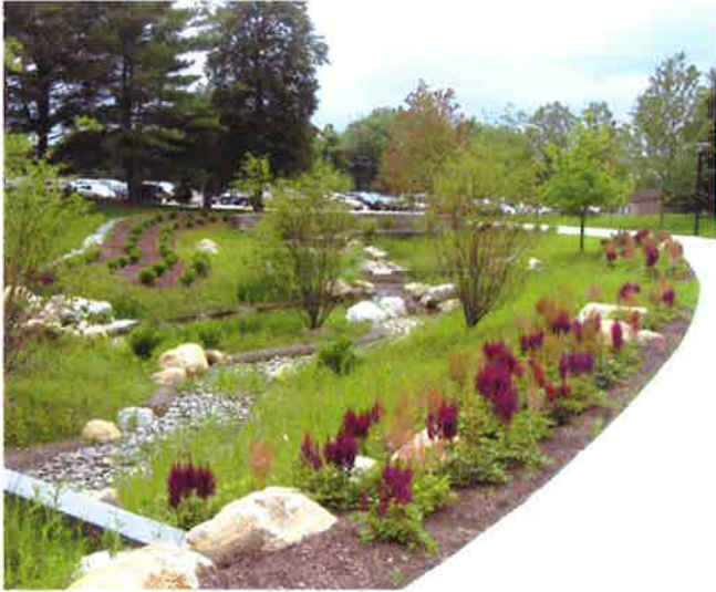
Stormwater bioretention planter
