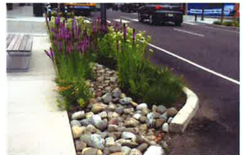
Stormwater bioretention planter
