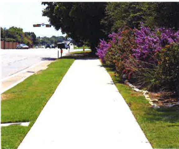
Sidewalk with grass buffer
