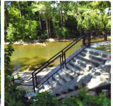
Steps with railing to river
