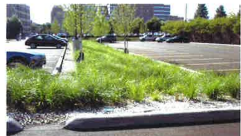
Stormwater bioretention planter
