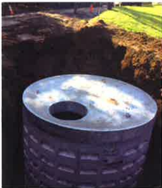
Dry Well Installation
