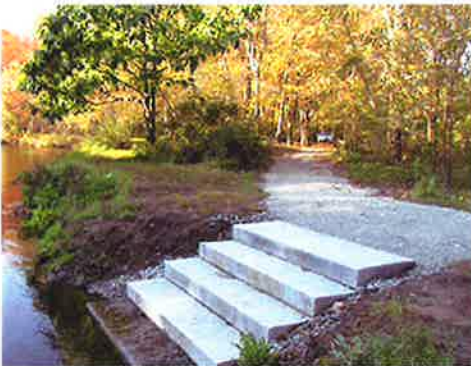
Concrete steps to river
