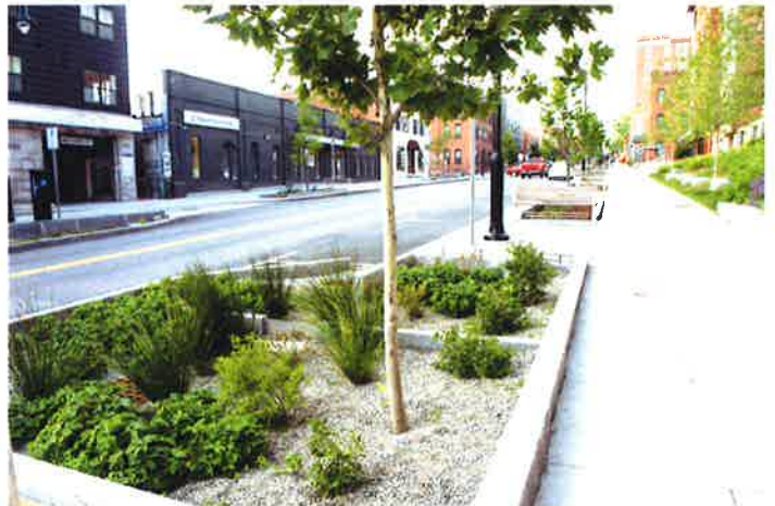
Rain garden sidewalk planters
