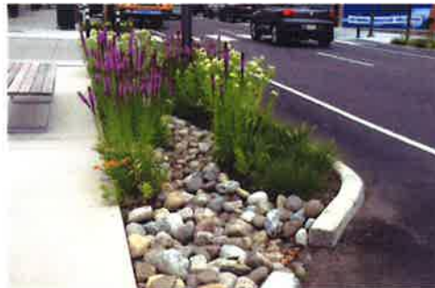
Stormwater bioretention planter
