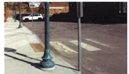
East Street Crosswalk
