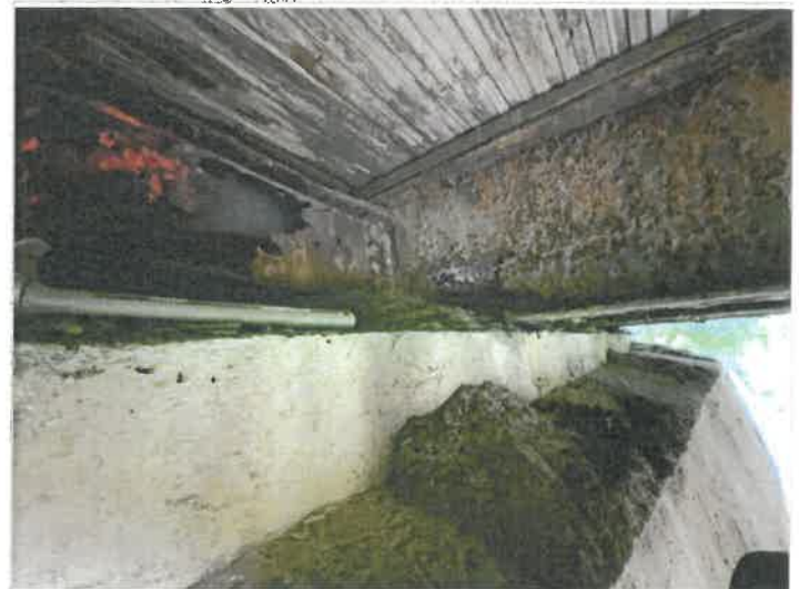
Abutment 2 beam ends
