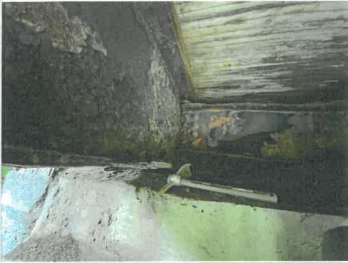
Beam 1 abutment 2 end
