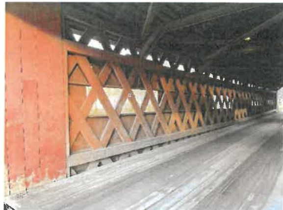
North Truss Looking East
