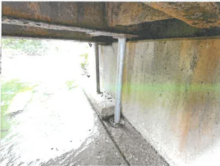
Beam 2 abutment 2 end
