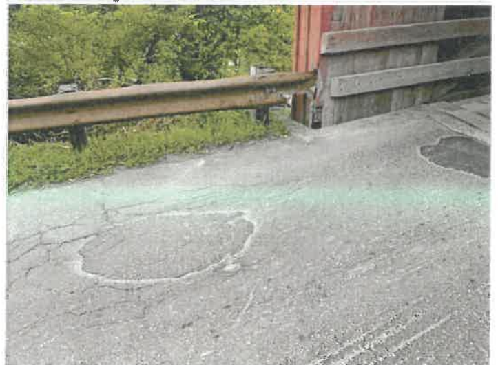
Abutment 2 transition rail
