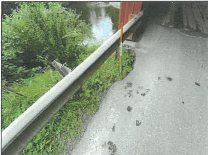
Upstream abutment 1 shoulder area
