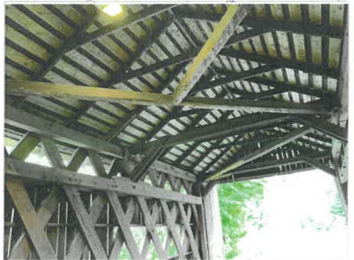
Lateral cross bracing
