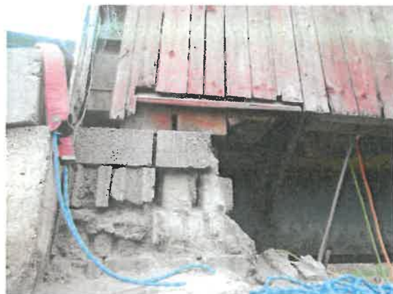
Timber Bearing and CMU Blocks
