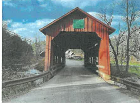
South Portal Looking North
