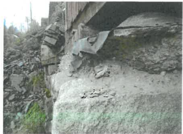
West Abutment Beam Seat
