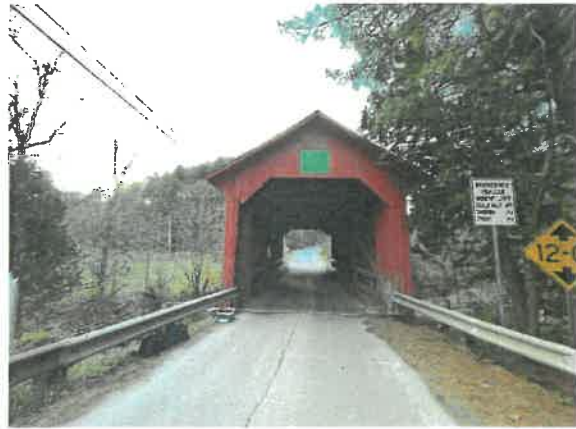
East Portal Looking West
