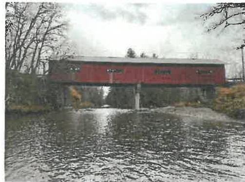
Downstream Elevation Looking South
