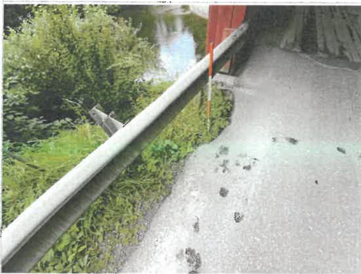
Upstream abutment 1 shoulder area
