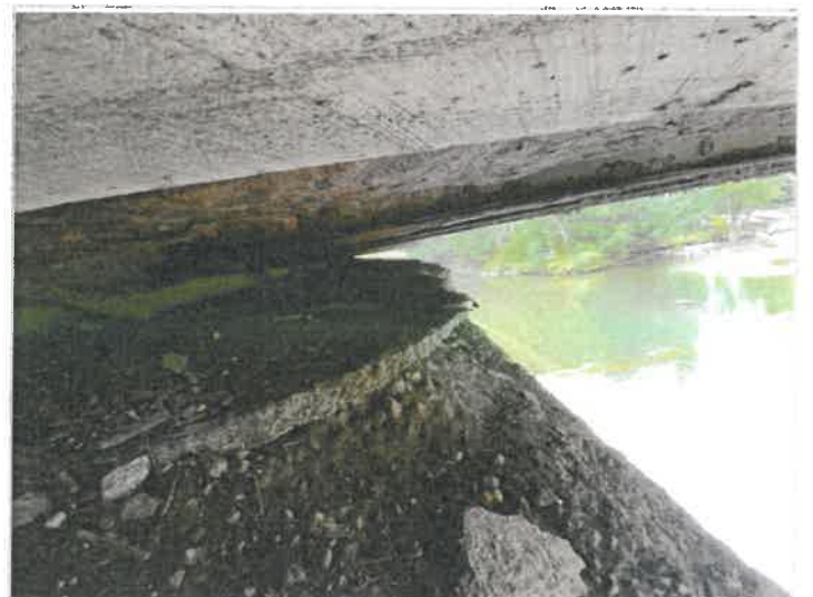
Abutment 1 beam ends
