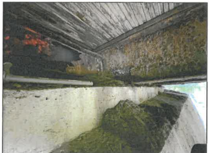
Abutment 2 beam ends
