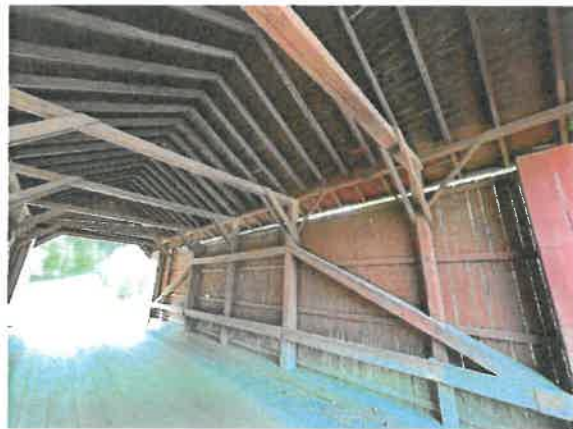
North Queenpost Truss
