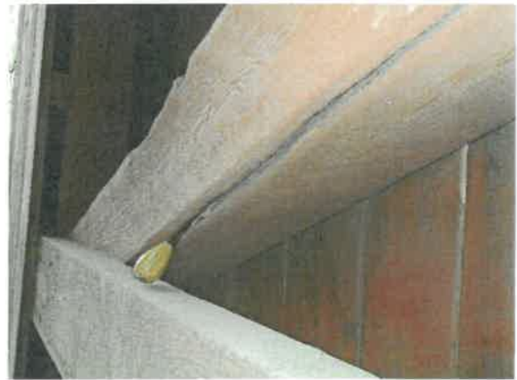
Southeast Diagonal Check at Bottom Chord
