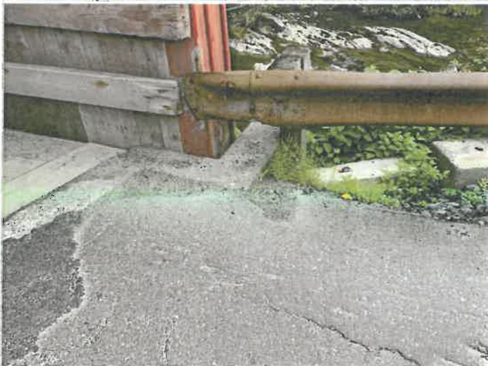
Abutment 2 transition rail
