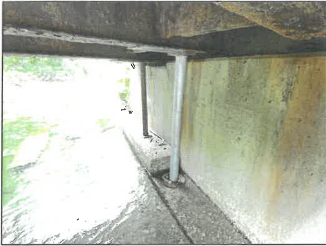
Abutment 2 beam ends
