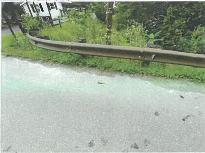
Downstream abutment 2 approach
