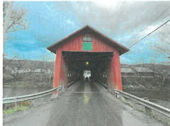
West Portal Looking East
