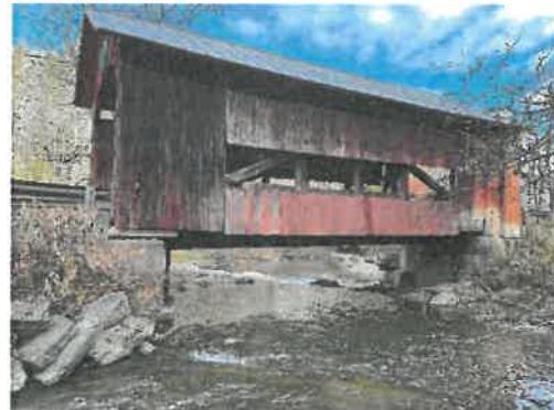
Upstream Elevation Looking East
