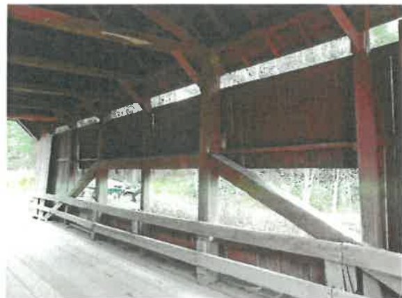
West Queenpost Truss
