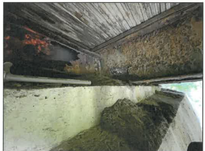
Abutment 2 beam ends
