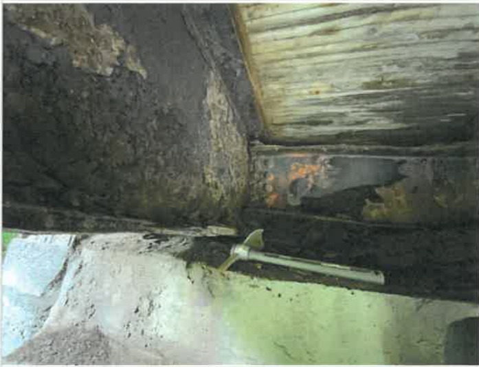
Beam 1 abutment 2 end
