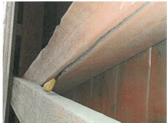
Southeast Diagonal Check at Bottom Chord
