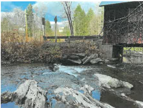
Upstream Channel with Exposed Bedrock
