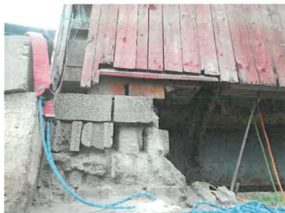
Timber Bearing and CMU Blocks
