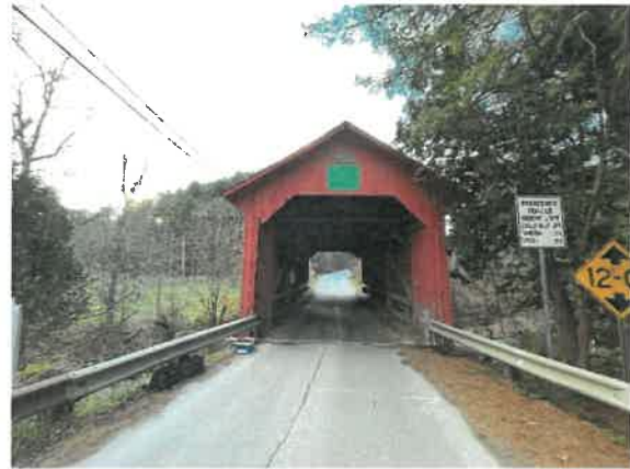
East Portal Looking West
