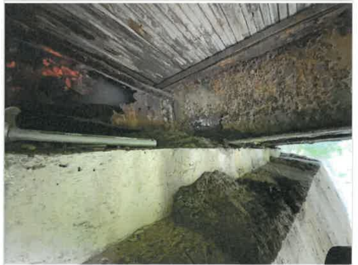
Abutment 2 beam ends
