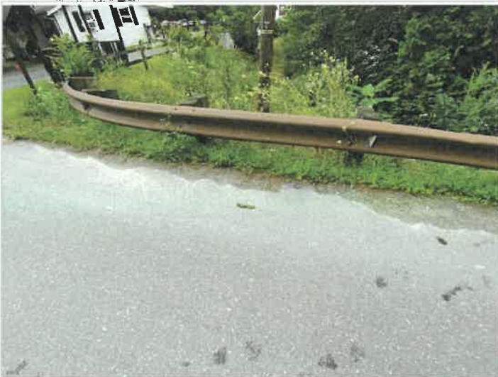
Downstream abutment 2 approach
