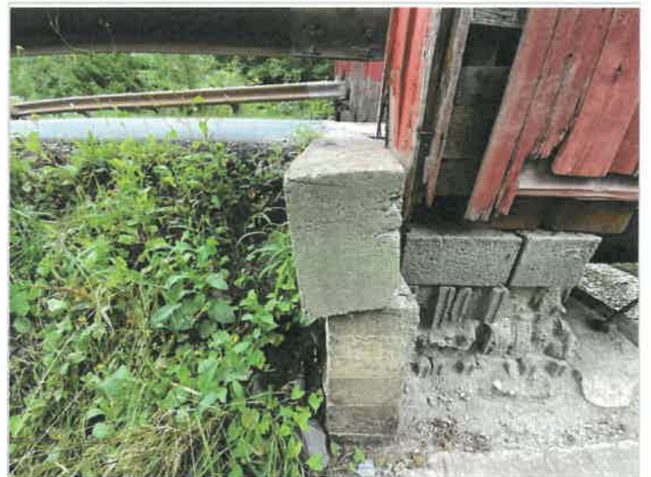
Abutment 1 backwall
