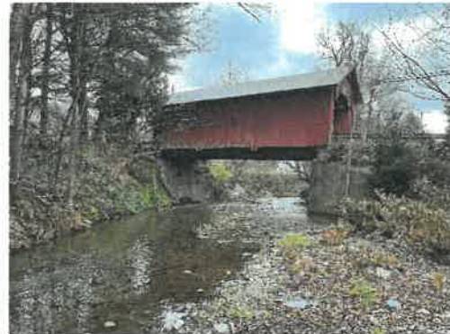
Upstream Elevation Looking South
