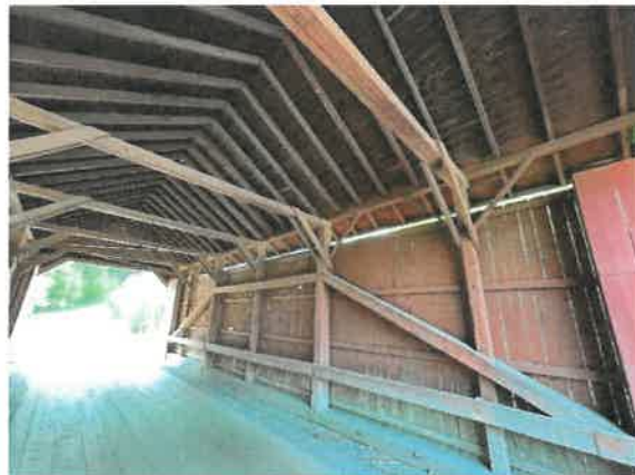
North Queenpost Truss
