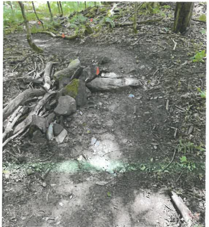
Portion of the new rerouted trail. The crew resurfaced though here and installed a couple stone steps
