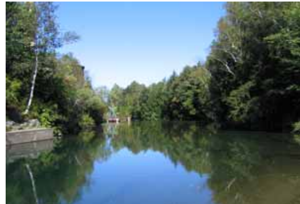
Figure 5.32: Impounded channel above Northfield Mills dam near Belknap Street
