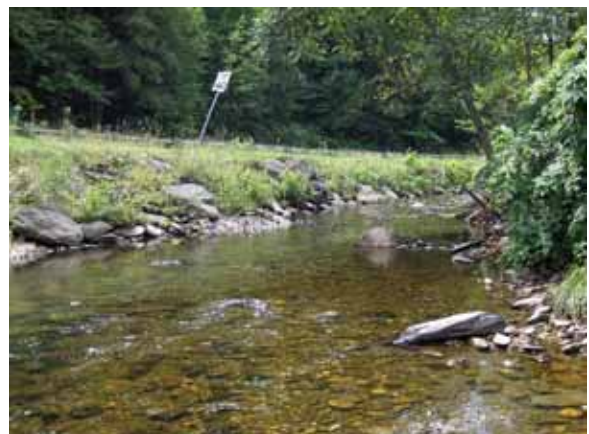
Figure 5.40: Straightened channel with no riparian buffer along Route 12A near Stony Brook Road
