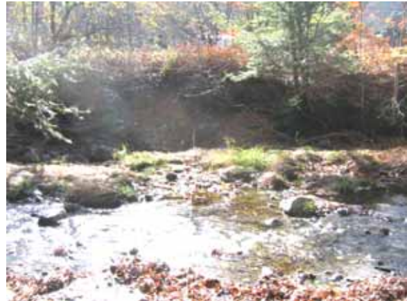
Figure 5.60: Incised channel and flood chute looking at south bank downstream of driveway bridge off Cox Brook Road below Jerry Road
