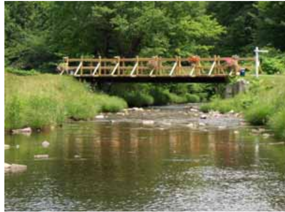
Figure 5.42: Straightened channel through golf course at Northfield Country Club with no riparian vegetation and bridge
