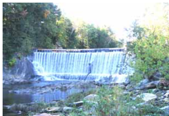
Figure 5.31: Northfield Mills hydroelectric dam near Belknap Street
