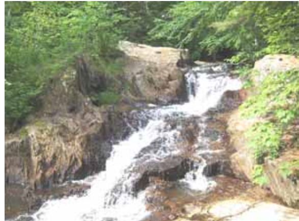
Figure 5.49: Grade control near Beaudette Road Bridge
