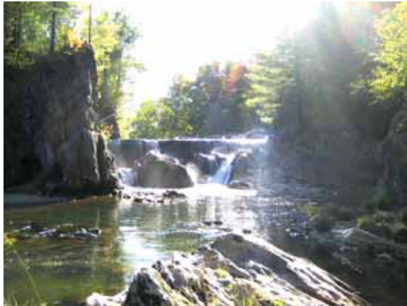
Figure 5.22: Dam and bedrock near MWT Products on Mill Street
