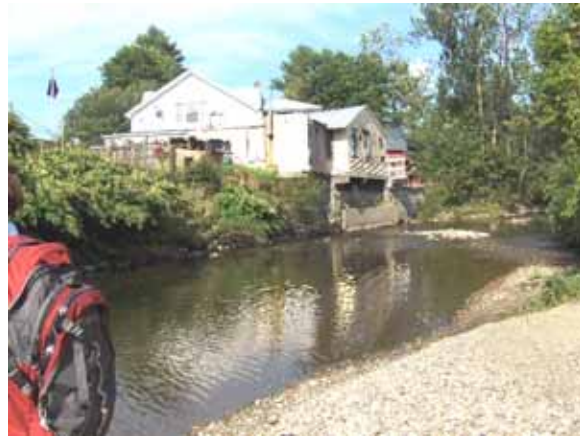
Figure 5.36: Houses built along Dog River on Water Street near intersection with Western Avenue
